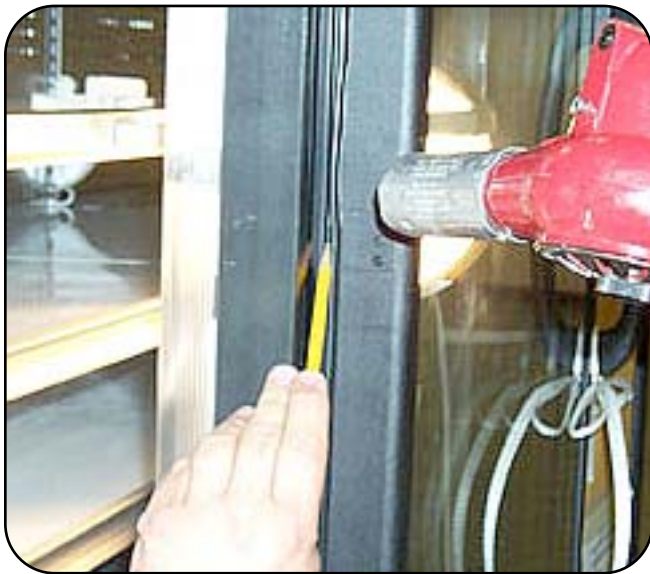
Figure 15. Pulling Gasket Into Place With a Pencil
